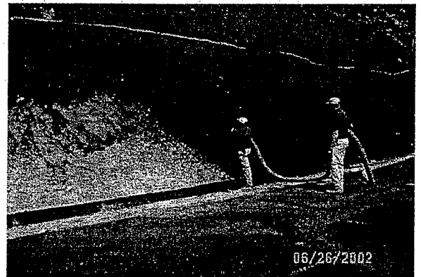
The contractor used a pneumatic blower to apply the compost.
